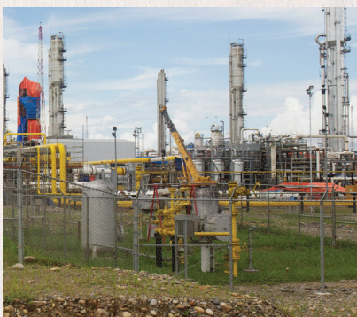
a natural gas power plant
